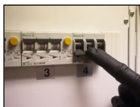
1. Turn of the power to the oil mist detector...
