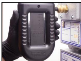
7. connect the U- tube manometer and adjust the
