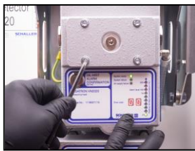
1. Unscrew the four bolts on the inspection cover...
