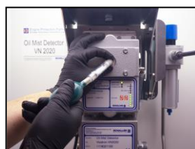
9. pump smoke until the oil mist alarm are realised....
