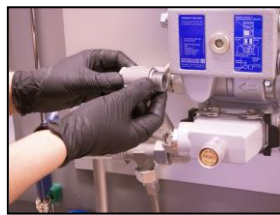
2. remove the pipe from oil mist detector...
