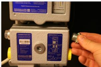
change the screw plug seal 1/2" (P/n.: 10209)...
