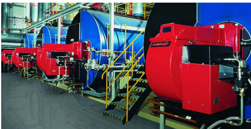
RGL70 dual fuel burners in a district heating centre
