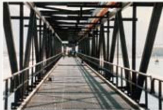
Offshore terminal, Fujairah
