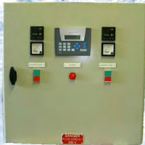
Compressor starter- and control panel
